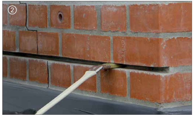
Fuge reinigen | Nettoyer le joint
